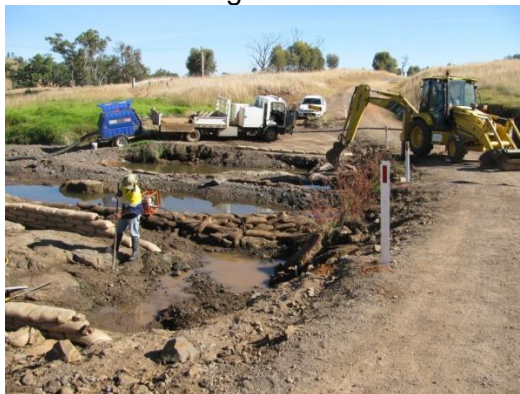
Replacement of flood damaged causeway over Garrawilla Creek on Wyuna Road.
